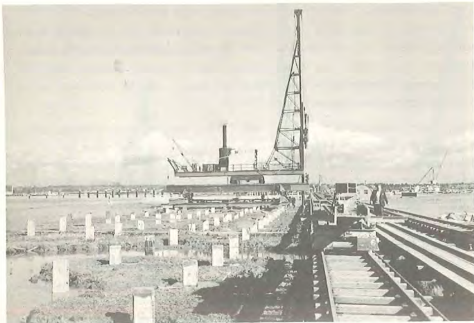
Fig. 62 Cantileverrambuk (57)
